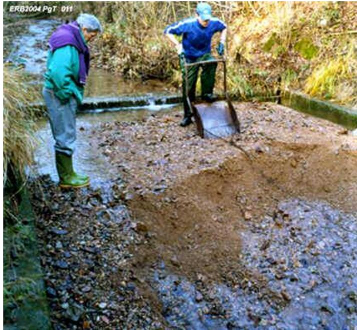
The sedimentary station at the time of material removal (upstream view)
